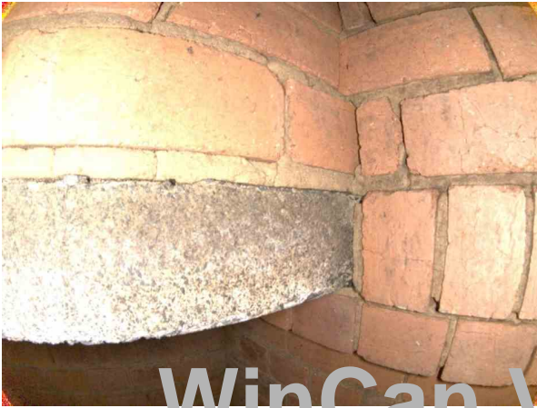
1, , 0.64 All or part of the mortar from masonry is missing, 5mm from 5 o'clock to 10 o'clock
