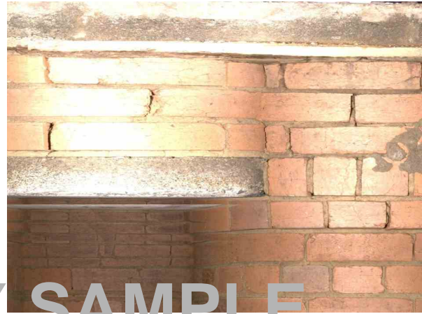
2, , 0.64 All or part of the mortar from masonry is missing, 5mm from 5 o'clock to 10 o'clock
