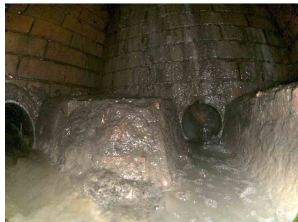
6, , 6.55 A conduit connecting to the maintenance structure, circular, incoming., Ht/Dia # 150mm at 6 o'clock
